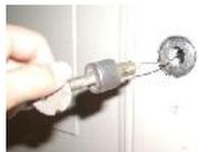
A door mounted release is available for releasing the door from outside.
