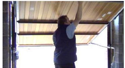
Fix the second 'U' bracket half way along the rail. This time you must use the two plastic rail clamps because the J bracket passes this point
