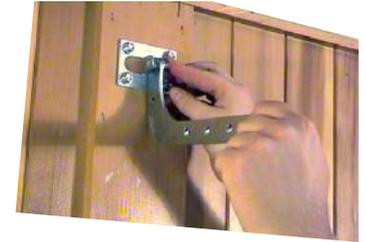
Fit the 'J' bar to the door bracket with the cotter pin. Insert the split pin. Open one leg to secure it.
