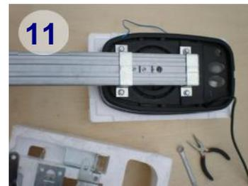
The roof hangers may also be fitted to the rail and motor head if you know the roof joist positions. Apply a finger of grease to the chain.
